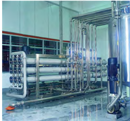
Fig. 12.37 Installation of spiral wound filter
